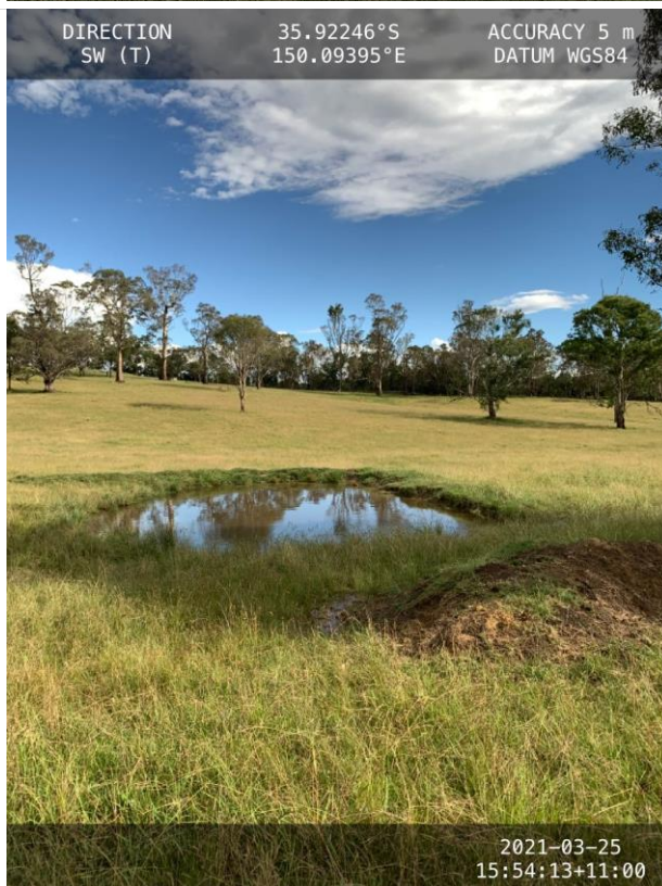
Photograph 4: Taken showing an example of one of the several dams across the site. Note the soil pushed to form a batter to create the dam.
